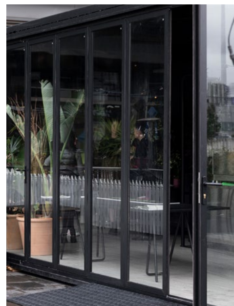
bi-folding glass doors on a track
