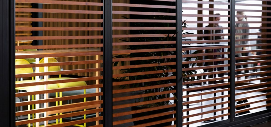
teak timber horizontal panels
